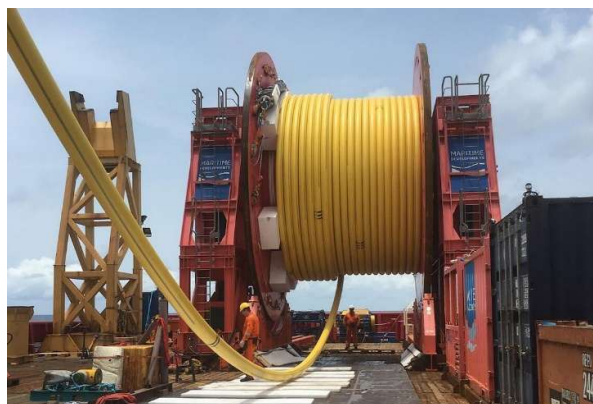
Figure 8 Cable being pulled from a reel [10]
